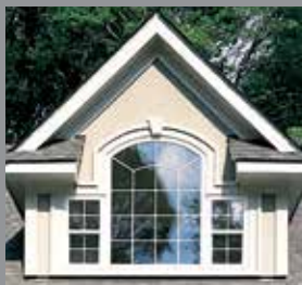
Under the eaves. A tall window like this fixed extended arch flanked by double-hungs can open up a top floor.
